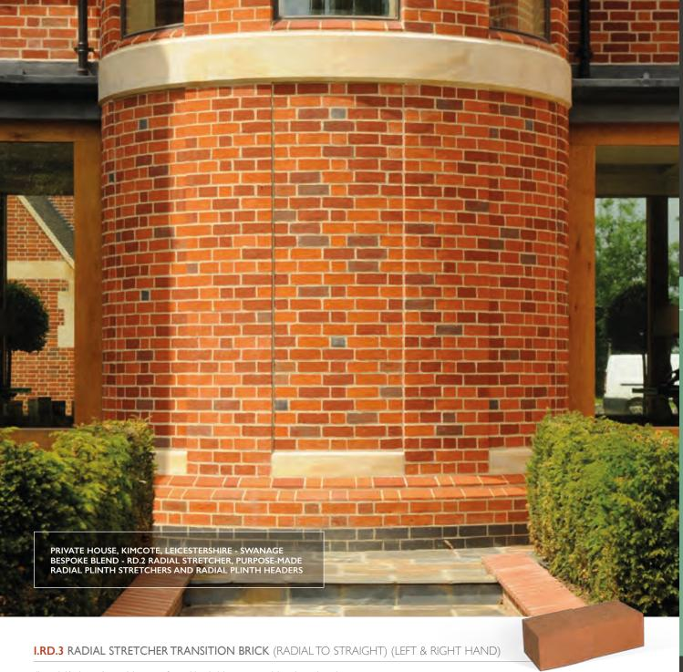
Ibstock Kevington's special range of transition bricks are essential at the point where curved brickwork changes to straight. \*Dimension A in types I.RD.3 is a segmental length.
